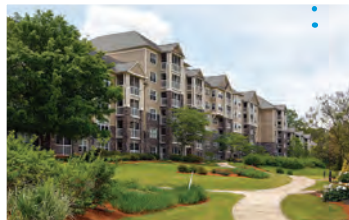
Lanier Village Estates Gainesville, GA
