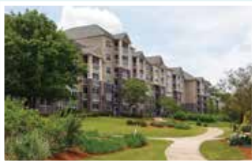
Lanier Village Estates Gainesville, GA
